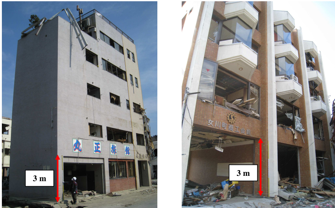
Figure 10 Damage found at the 4 th floor, says more than 12 m tsunami height
