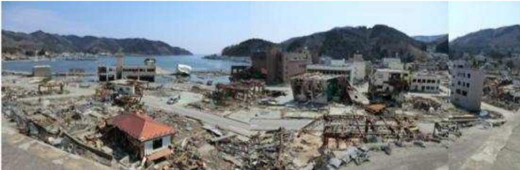
Figure 1. Almost entire city was washed away, only RC buildings stood still, however many of them failed from their pile foundations.
