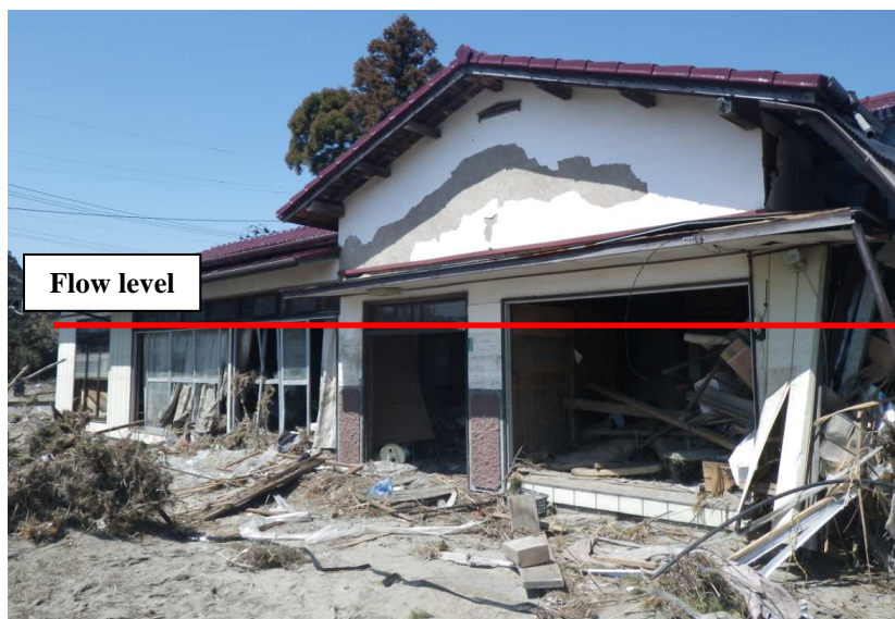
Type: one-story wood frame Function: residence house Flow depth: 1.77 m Damage: punched wall and damaged in some columns Location: Latitude = 37.984185 and Longitude = 140.893562
