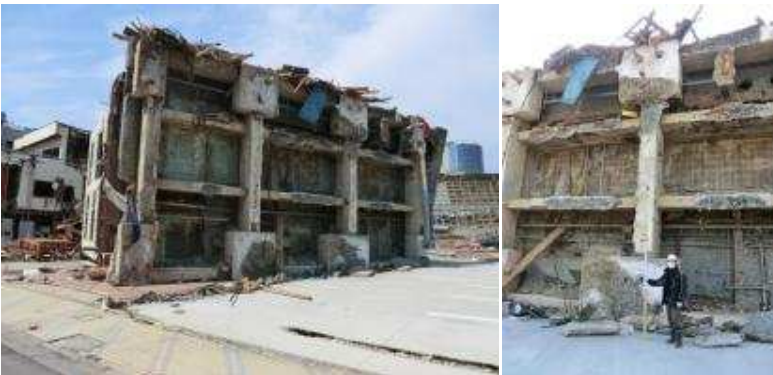
Figure 2. RC building fallen entirely, probably pile foundations failed and tsunami buoyancy force knocked the whole building down.
