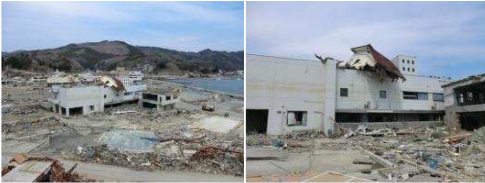
Figure 3. Tsunami inundation overtopped houses and buildings, wooden houses became floating debris.
