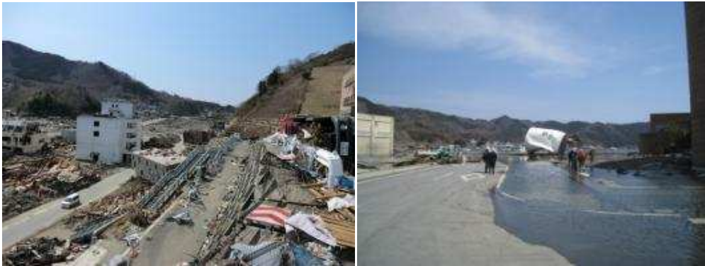
Figure 4. Inundation level went up to the hospital at the hill, even inundating the first floor. In the right picture sea level inland due to subsidence (aprox. 70cm)
