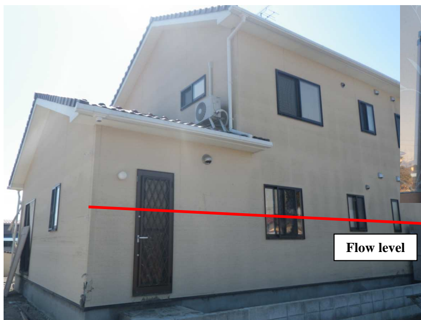
Type: two-story wood frame Function: residence house Flow depth: 1.94 m Damage: no structural damage Location: Latitude = 37.983961 and Longitude = 140.893869
