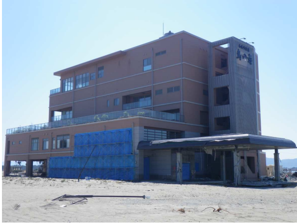
Type: six-story RC frame Function: Watari spa Tori no Umi hotel Flow depth: unknown (broken window glass until second floor) Damage: no structural damage Location: Latitude = 38.036667 and Longitude = 140.919089
