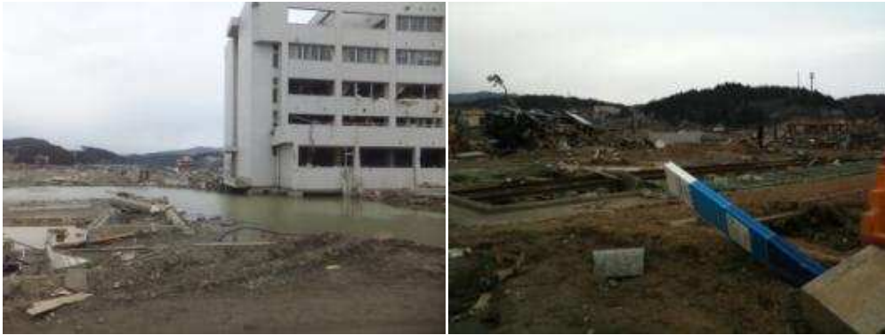
Figure 3 Scour on foundations and other structures like tsunami poles (monument in the right picture) resulted on structural damages.
