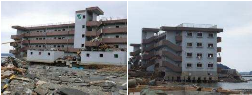
Figure 2. Tsunami Evacuation Buildings resist tsunami impact and saved lives, on the contrary other shelters like a school was washed away.
