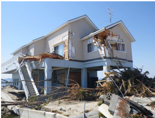
Type: two-story wood frame with RC column Function: Residence house Flow depth: 8.6 m Damage: wall due to tree debris and severe scouring at foundation Location: Latitude = 38.036968 and Longitude = 140.917572
