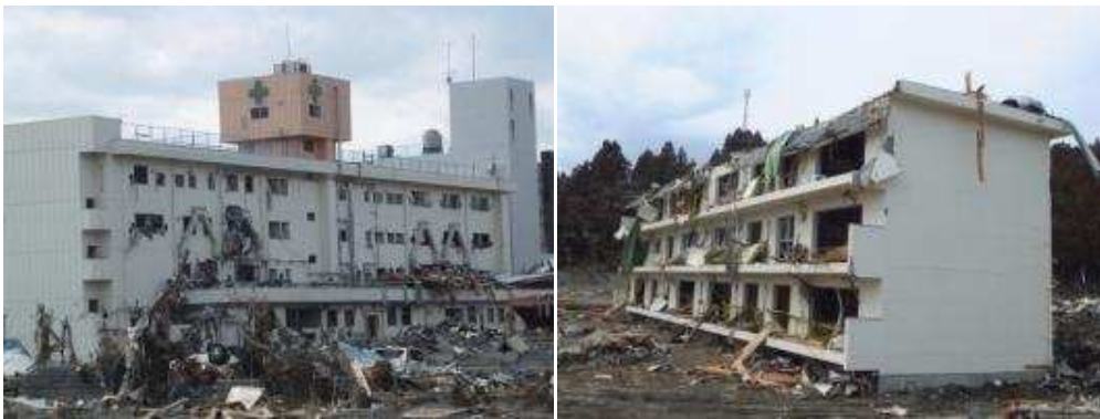
Figure 1 Several RC buildings resist the tsunami impact, however almost all of them were inundated at all its floors.
