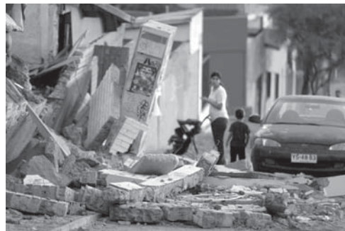
Fig. 5 Collapsed home in Iquique (ABC News)
