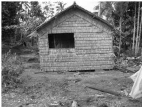
Photo 3.4.11.1 High-floored house in Fig. 3.4.11.2 moved by the tsunami
