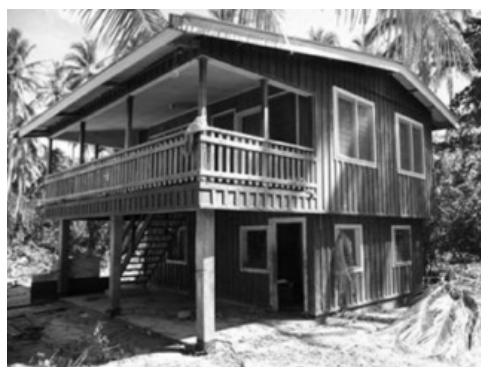
Photo 3.1.3.1 House that withstood 2 m of tsunami inundation
