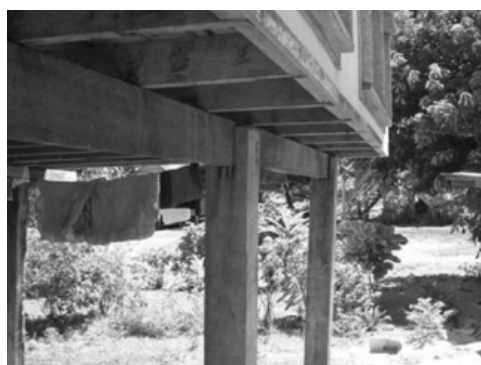
Photo 3.4.2.1 Connection between piers and floor in Sambora.
