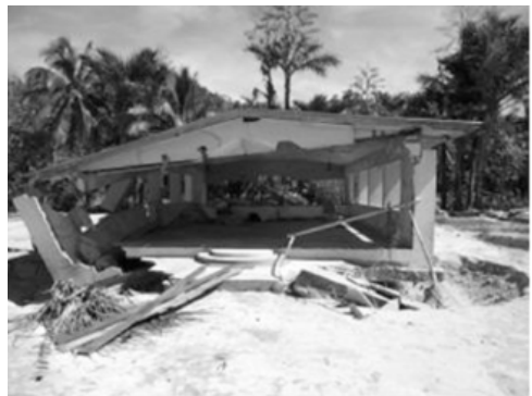
Photo 3.1.3.4 Erosion of foundation of structure in New Manra
