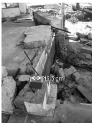
Photo 3.1.2.4 Broken front section of the damaged church
