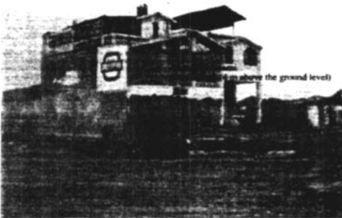
Figure 6 Hotel building struck by the tsunami at La Punta.
