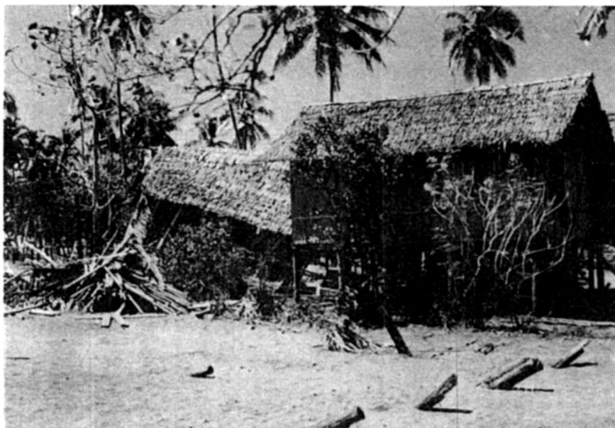
Photo 8 Damaged houses in the left. A house with low floor was swept away. A sheltered house (right) with high floor remains without severe damage
