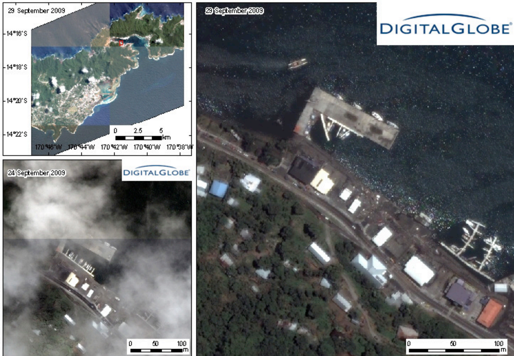
Damage in a small harbor in Pago Pago.
